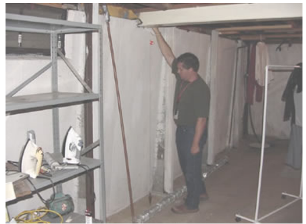
Inward deflection of a basement wall and pilasters. The plumb-bob reveals 9 inches of inward displacement. U.S. Army Corps of Engineers Photo Click Image to Enlarge
